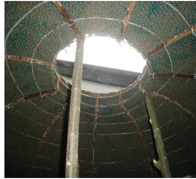
Various stages of the building process of an On-Surface/Above-Surface RWH Unit at Idamelanda, Left – concreted base and wire mesh reinforcement, Middle and Right: Application of mortar to roof. Photo Credits: Janaki Chandimala, 2008.
