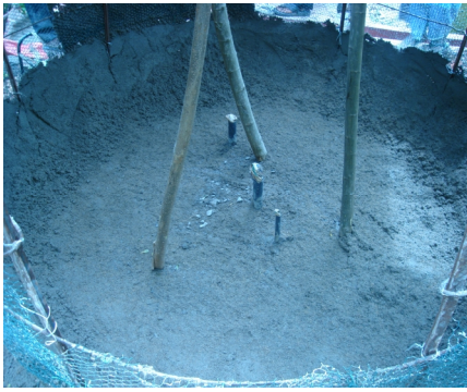
Various stages of the building process of an On-Surface/Above-Surface RWH Unit at Idamelanda, Left – concreted base and wire mesh reinforcement, Middle and Right: Application of mortar to roof. Photo Credits: Janaki Chandimala, 2008.
