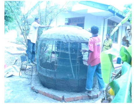
Various stages of the building process of an On-Surface/Above-Surface RWH Unit at Idamelanda, Left – concreted base and wire mesh reinforcement, Middle and Right: Application of mortar to roof. Photo Credits: Janaki Chandimala, 2008.
